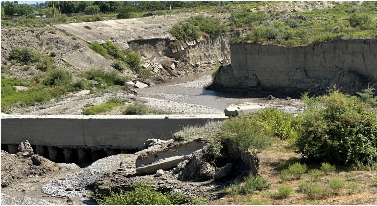
Figure 1. Opening of guard rail of "Baku-Khachmaz" road bridge by washing.
