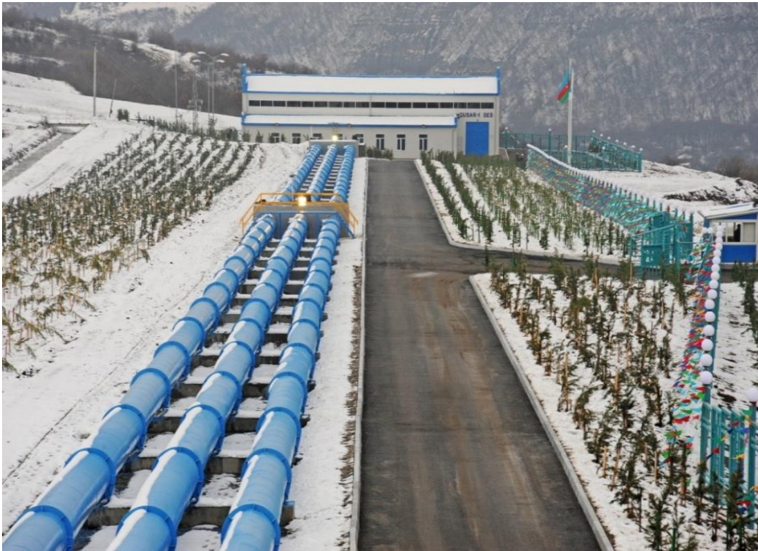
Fig.2 "Gusar-1" small HPP on the Gusar tributary channel
