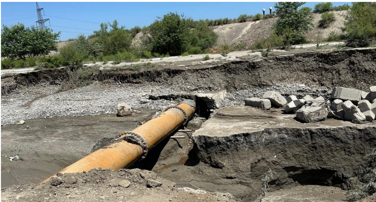
Figure 2. Opening by washing the "Shollar-Baku" aqueduct crossing from the Velvele river
