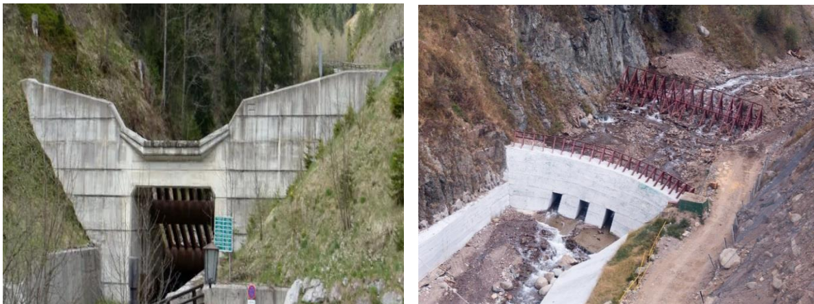
Figure 12. Combined flood catchment devices
