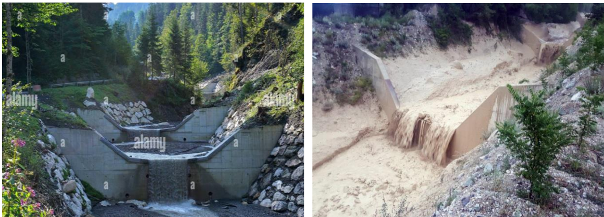
Figure 11. Sequential threshold flood dampers along the channel
