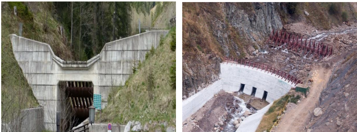
Figure 12. Combined flood catchment devices
