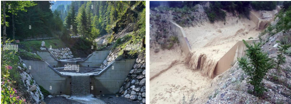
Figure 11. Sequential threshold flood dampers along the channel
