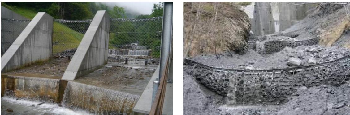
Figure 10. A flood catchment device made of steel mesh
