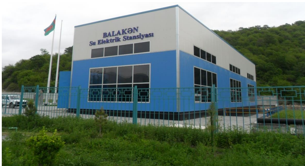
Fig.3 "Balaken-1" small hydropower station on the Balaken river
